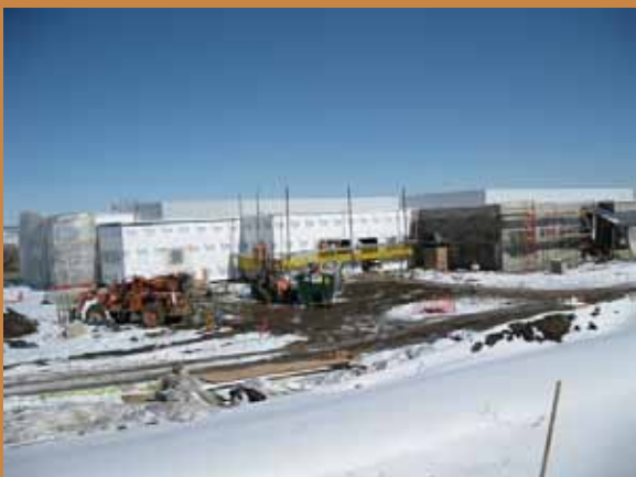
View of construction site, February 2010
